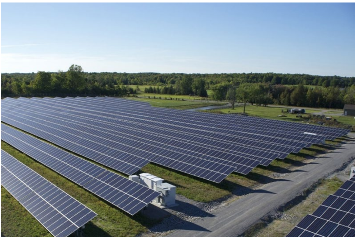
Image 4.2: Typical Fixed Panels (with Conversion Unit/Inverter)
